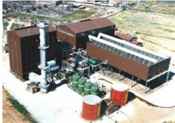
The gas, with main combustible constituents of CO and H<sub>2</sub>, is fed from the furnaces via wet scrubbers to a custom designed water tube boiler. The resulting high pressure steam is then passed through a fully condensing steam turbine attached to a 50 MWe generator. The steam is condensed in an air cooled condenser rather than a water cooled system in order to conserve water.
